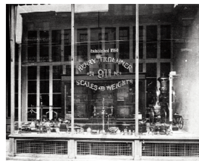
Troemner Storefront, 911 Arch Street, Philadelphia, Pennsylvania
